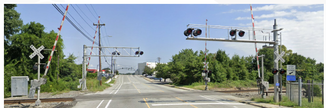
The Project will leverage STIP Project P-5747 to create a multimodal grade separated railroad crossing at S English St
